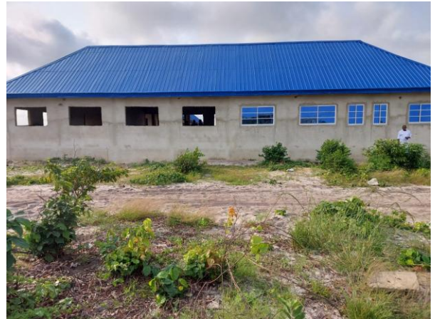
Fixing of Windows on the Block of 8 Classrooms
