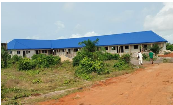
Front distant view of the complete block of 8 Classrooms
