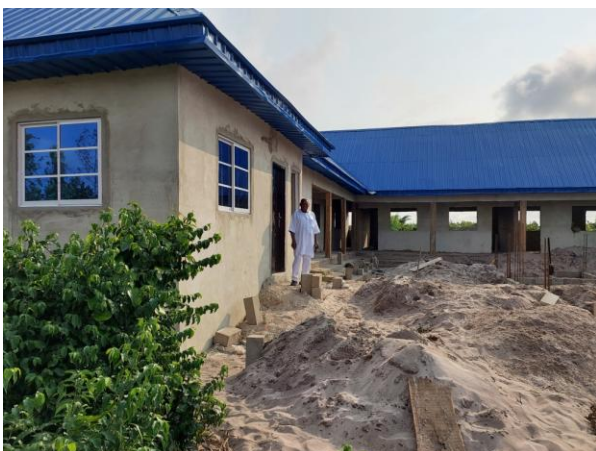
First completed stage - Block of 8 Classrooms
